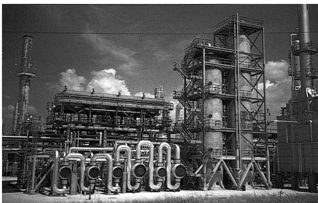
Fig.3 LB-52 is a must for plant construction
